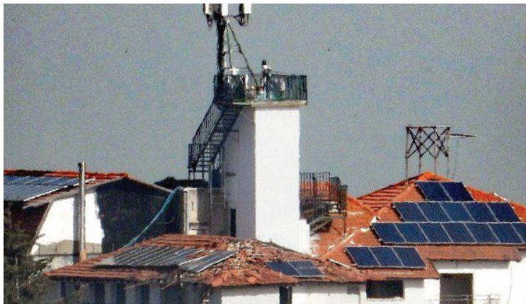
Damaged Israeli houses in Metula as seen from Lebanon | Source: web.telegram.org/k/#@eretz
