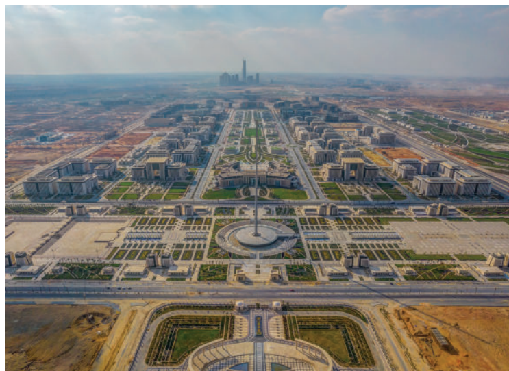
The New Administrative Capital under construction / Photograph: Shutterstock.com
