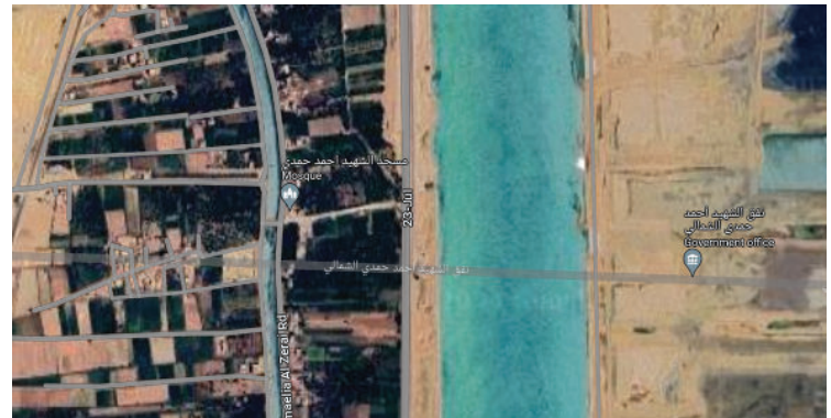
The Ahmad Hamadi Tunnel, a vehicular tunnel under the Suez Canal / Photo: Google Maps
